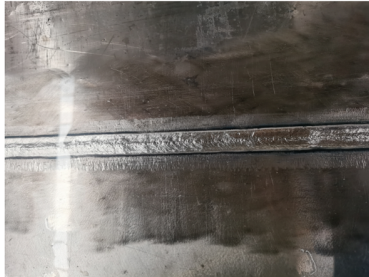
图 2 焊缝外观形貌 Fig.2 The appearance of the weld
